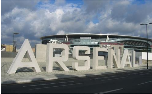
Figure 2: These letters are reportedly capable of withstanding the impact of a 7-tonne lorry driven at 50mph.
