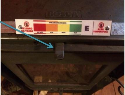
Damper's setting recording device
