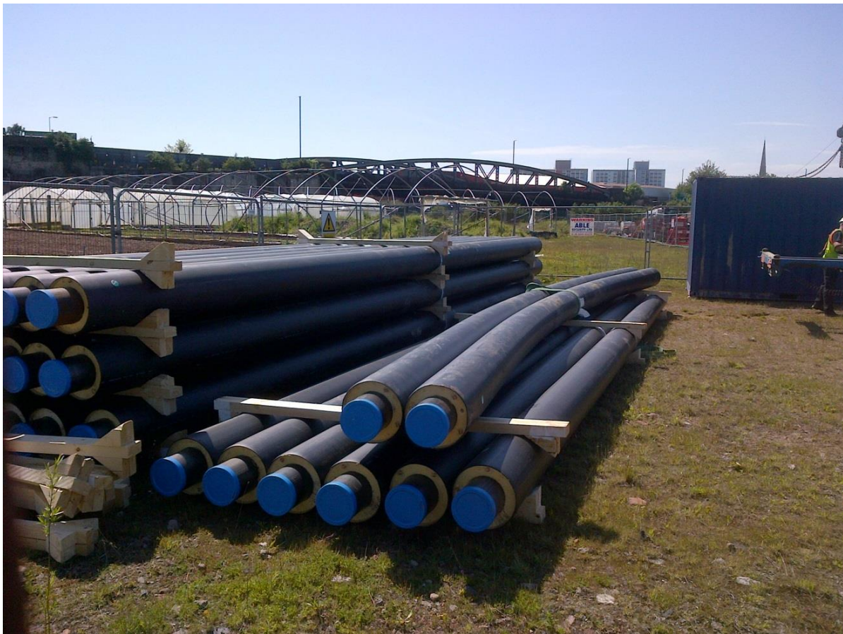
Figure 4: heat network pipework ready to be installed in Bristol
