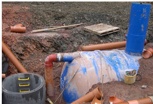
The underground storage tank for the RWH system
