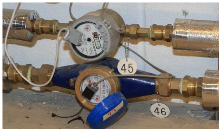
Monitoring equipment for the RWH system - meters (left) and water quality sampling point (right)
