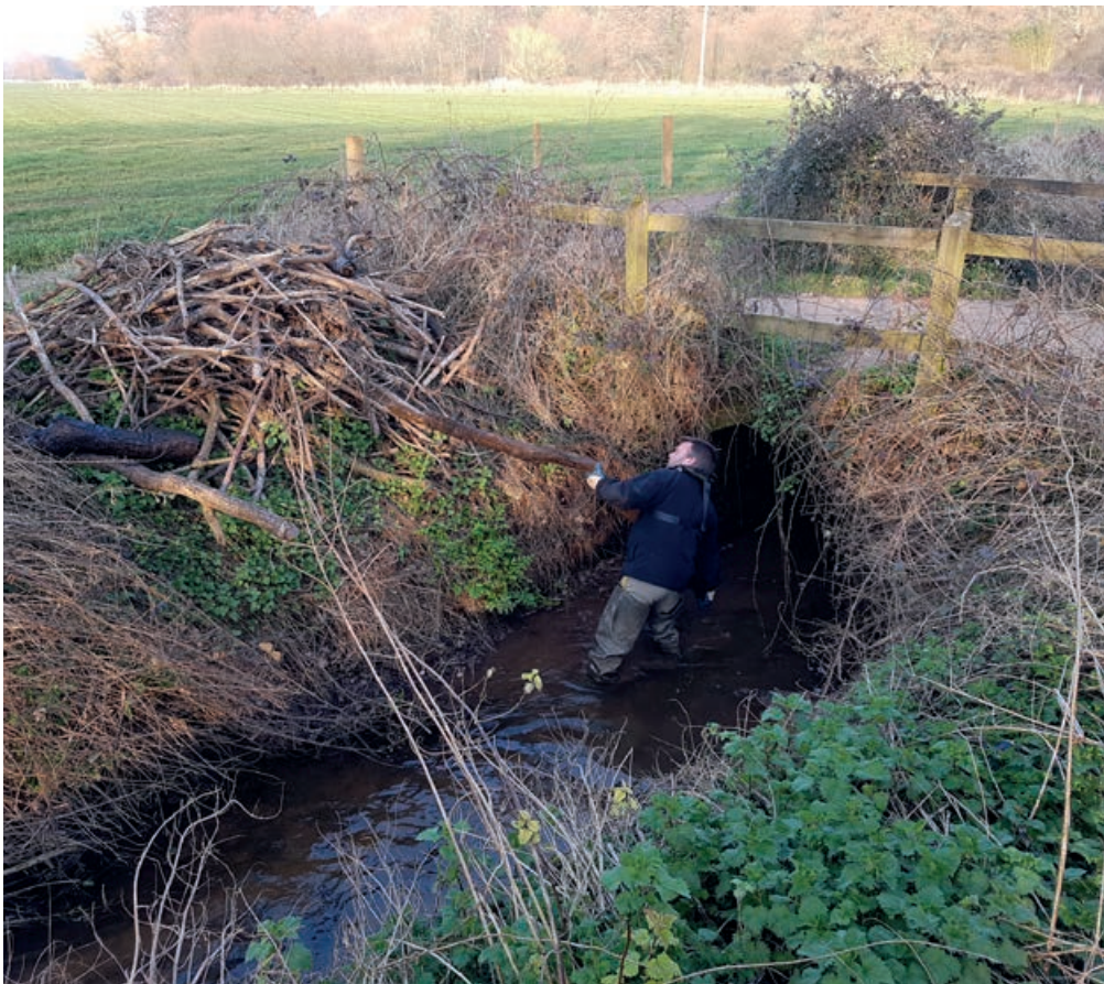
← ROBT Staff clearing a blocked culvert
