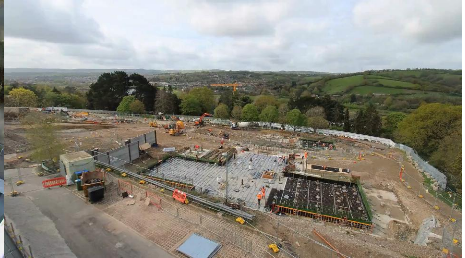
Construction of GH Block at West Park
